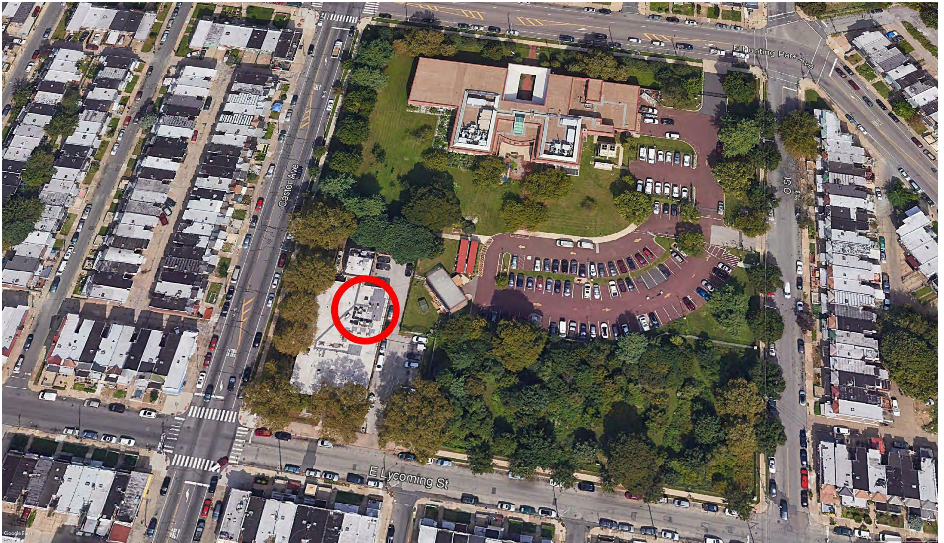
Figure 3 – LAB North Aerial View
