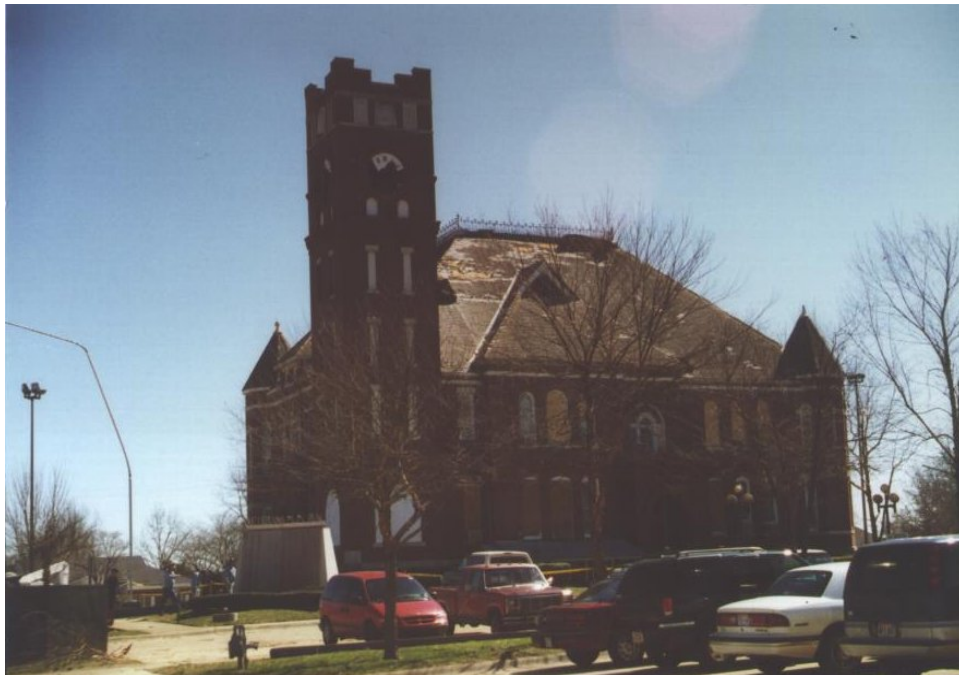
IB: DOD 6: Uplift of light-weight roof deck and insulation; significant loss of roofing material (>20%)
