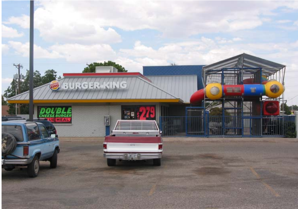
SRP: Hip roof, metal panel roof, wood trusses and stud walls, metal or vinyl siding
