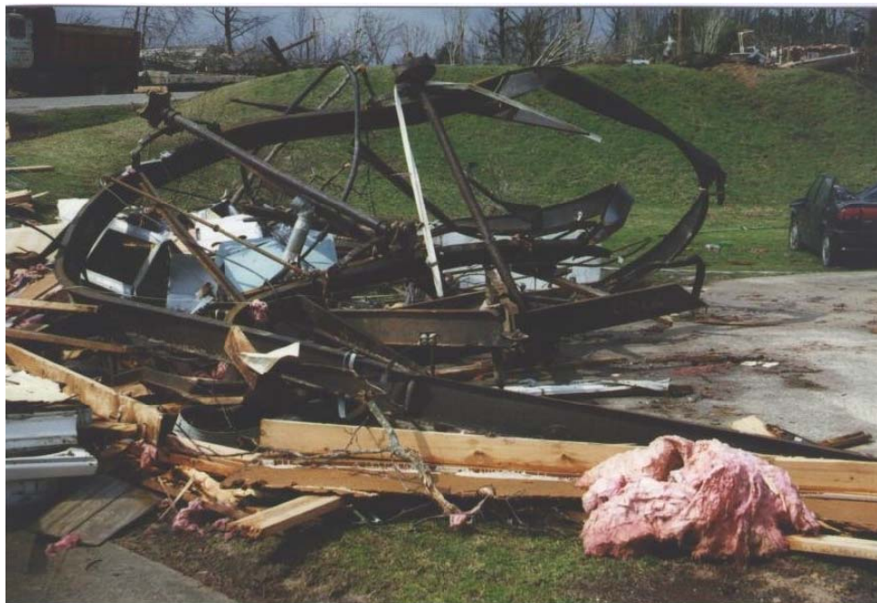
MHDW: DOD 11: Undercarriage separates from floor; rolls and tumbles, badly bent
