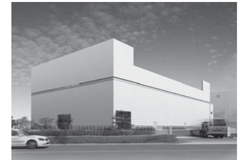
図10 燃料化施設外観図 Fig.10 View of Bio-Fuel Conversion Plant.
