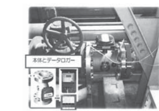
図14 自動水分計の設置状況 Fig.14 State of installation of automatic water content meter
