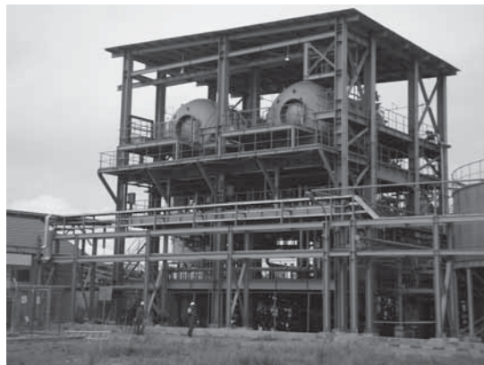
Fig.6 Filter building with two BOKELA HiBar disc filters (70m² each) for red mud filtration in an Indonesian Alumina refinery - TSK was EPC for this Alumina refinery with BOKELA as supplier of the complete filtration equipment.
