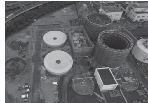
図1 消化タンク建設状況 Fig.1 Under construction of digestion tank
