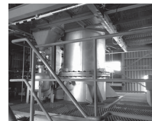
図7 過給式流動炉(フリーボード部) Fig.7 Photo of Fluidized Bed Incinerator with turbocharger(freeboard)
