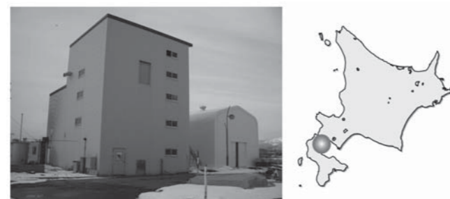
図4 実証設備建屋外観および長万部の位置 Fig.4 Photo and location of the pilot plant at Osyamanbe, Hokkaido, Japan
