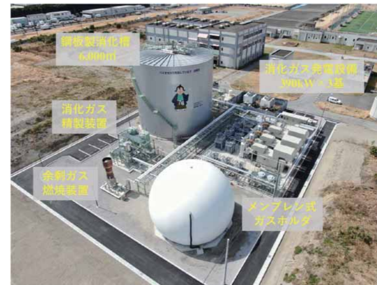
図5 完工後施設の外観機 Fig.5 Appearance of completed facilities
