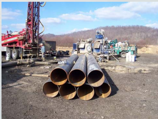
Surface Casing Rig
