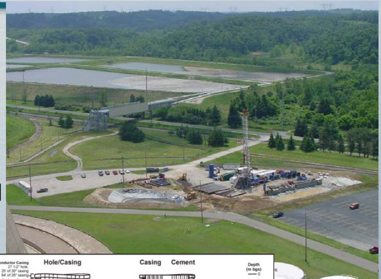
Drilling Test Well
