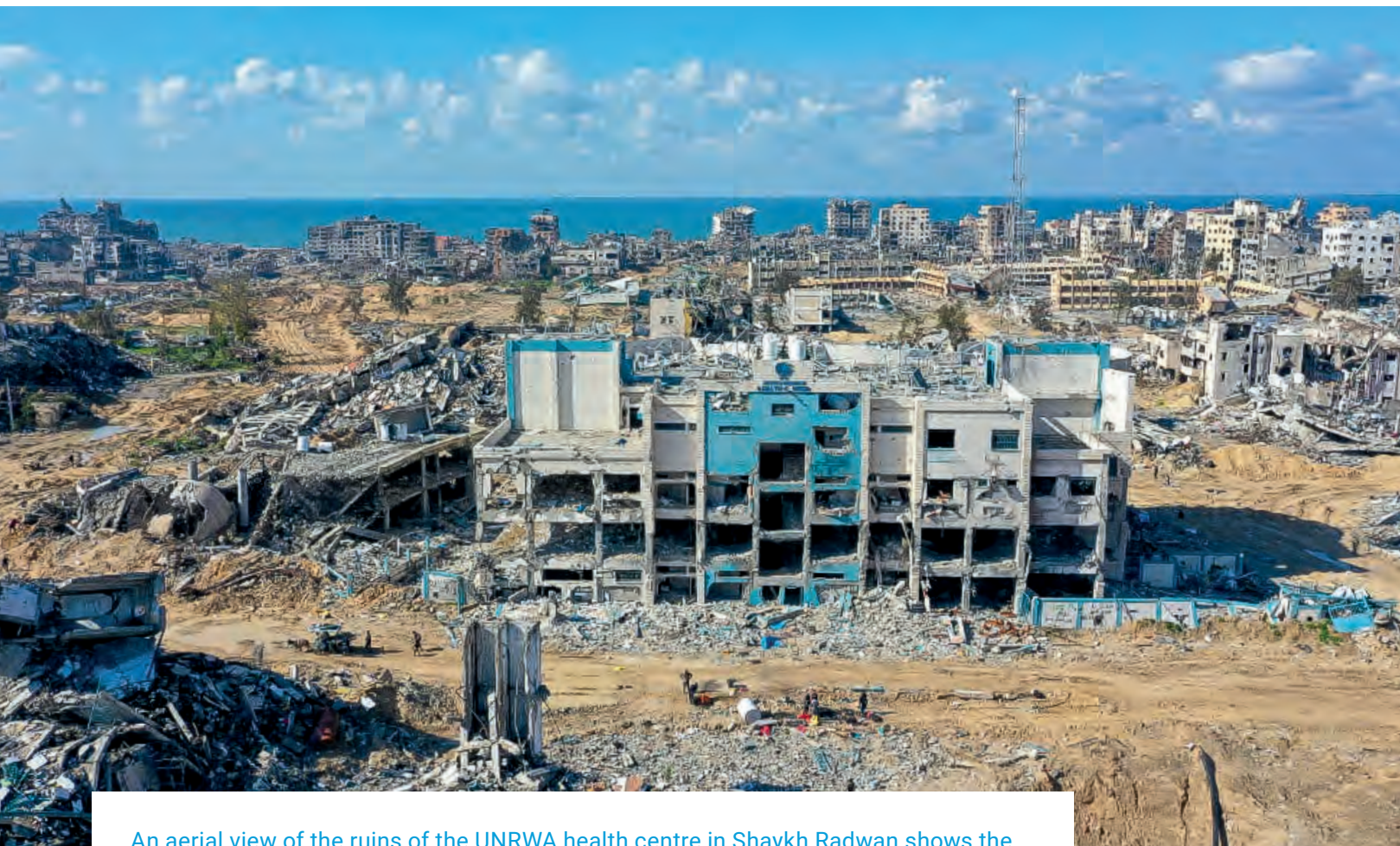
An aerial view of the ruins of the UNRWA health centre in Shaykh Radwan shows the extent of widespread destruction in the Gaza Strip since October 2023.
