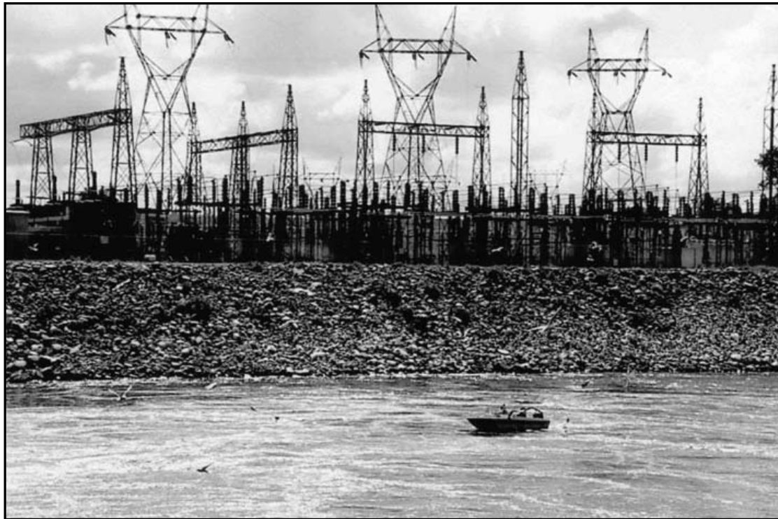
Figure 6-30: The switchyard at Garrison Dam. Source: David P. Billington.
