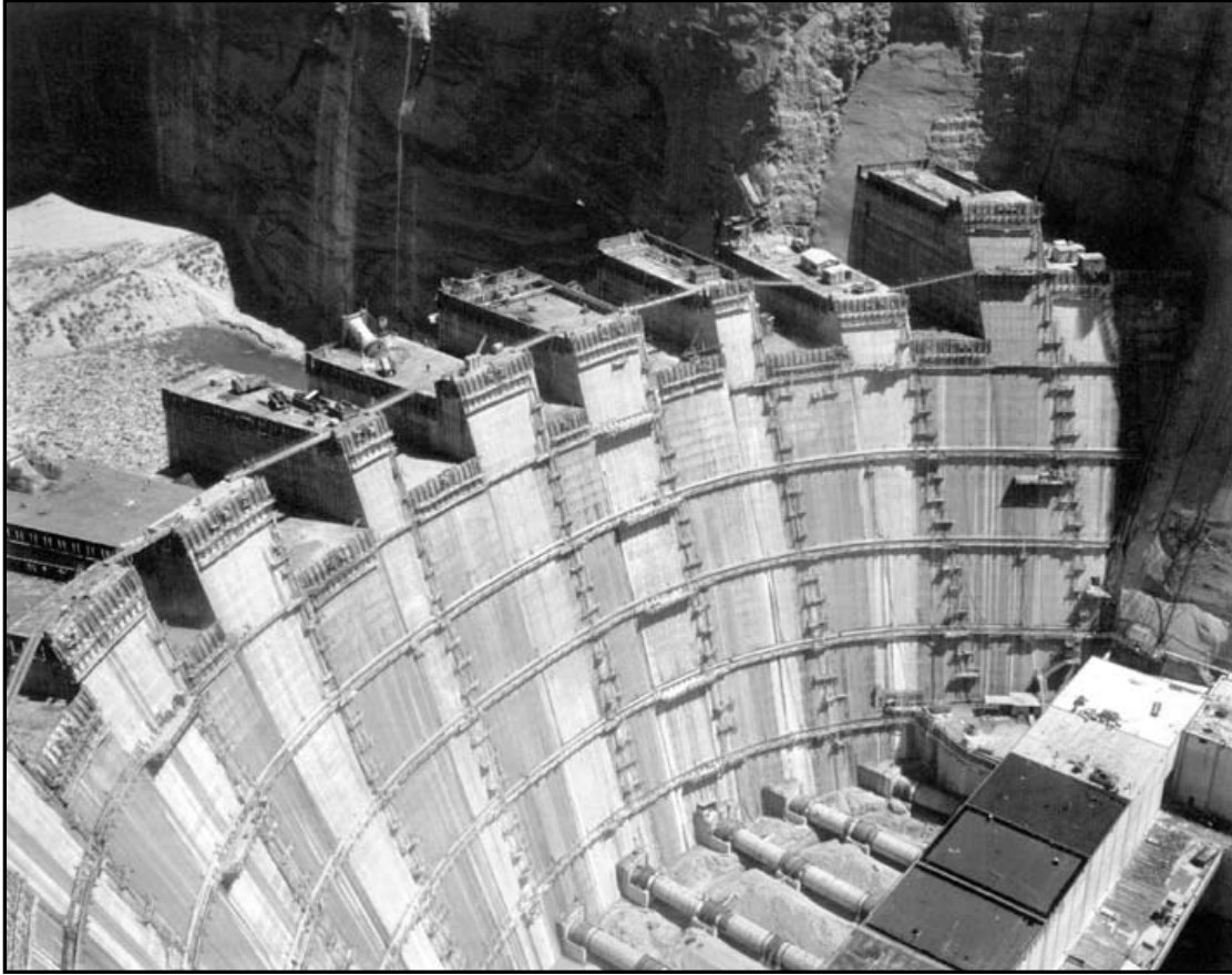
Figure 4-18: Glen Canyon Dam under construction on August 10, 1962. Source: Bureau of Reclamation
