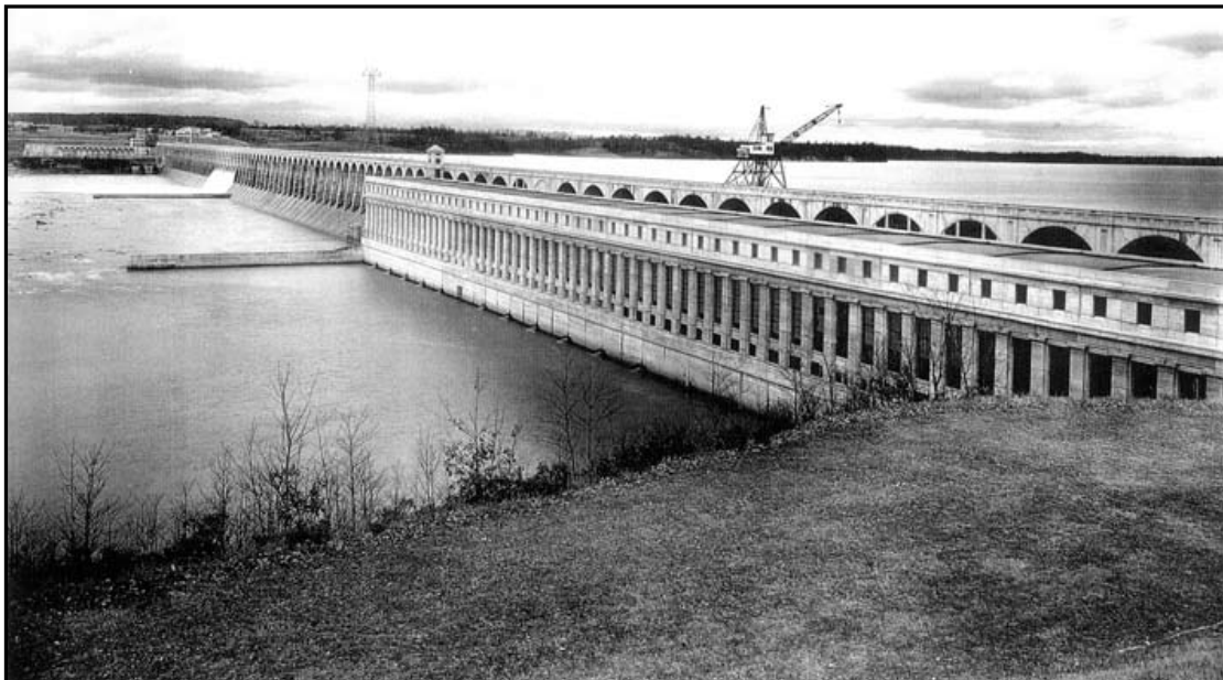
Figure: 3-8: Wilson Dam at Muscle Shoals on the Tennessee River was constructed under contract by the U. S. Army Corps of Engineers. Source: U.S. Army Corps of Engineers.
