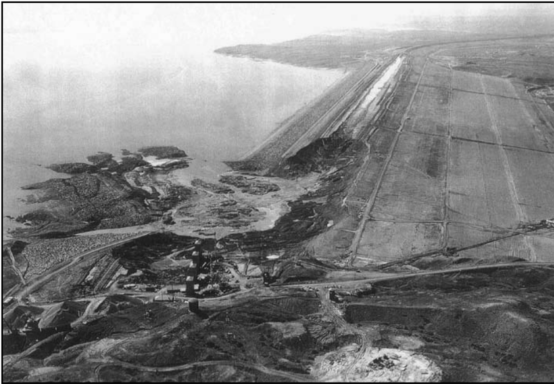
Figure 6-16: On September 22, 1938, a 5,000,000 cubic yard slide occurred on the upstream embankment of Fort Peck Dam. Source: Records of the U.S. Army Corps of Engineers, Record Group 77, National Archives and Records Administration, College Park, Maryland.
