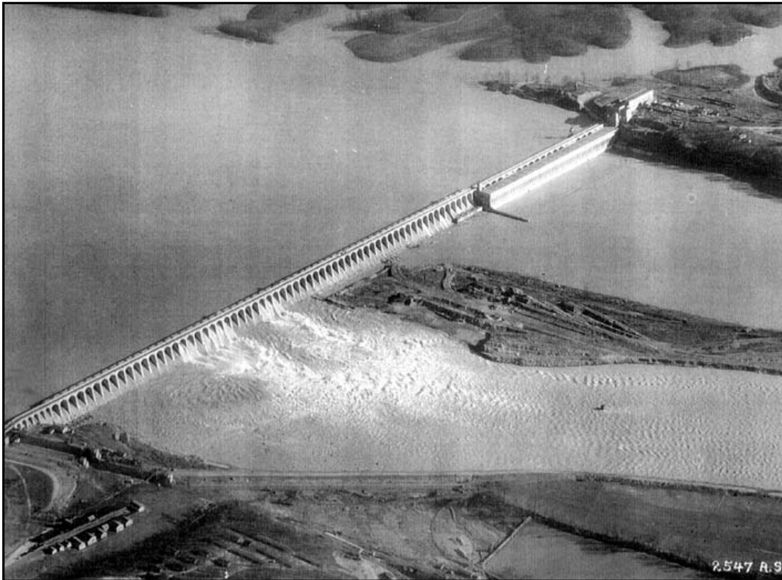
Figure 3-9: On July 13, 1923, open gates on the north end of Wilson Dam produced turbulent flow. Source: U.S. Army Corps of Engineers.
