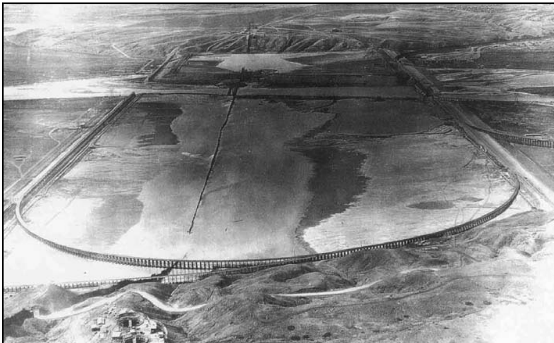
Figure 6-6: This September 12, 1935, aerial shows the entire hydraulic fill area of Fort Peck Dam, including trestles for dumping gravel and rock in the toes of the dam. Source: Records of the U.S. Army Corps of Engineers, Record Group 77, National Archives and Records Administration, College Park, Maryland.
