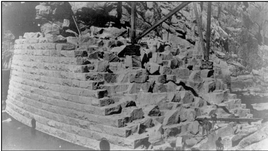
Figure 2-7: Pathfinder Dam was constructed with huge blocks of stone. Source: Bureau of Reclamation
