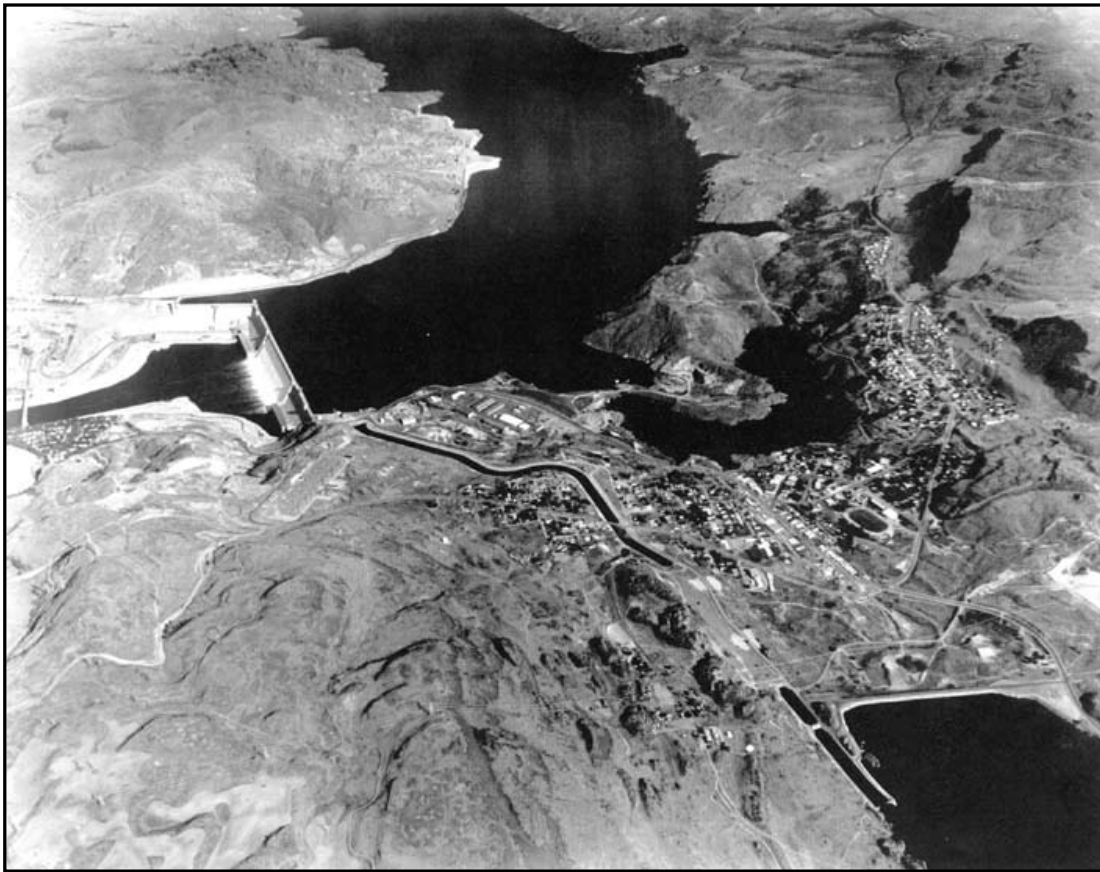
Figure 5-21: Grand Coulee Dam on the Columbia River, the feeder canal from the Grand Coulee Pump-Generating Plant outlet into Banks Lake (lower right). Banks Lake provides initial storage for water to be delivered to the Columbia Basin Project for irrigation of over 670,000 acres. Source: Bureau of Reclamation.
