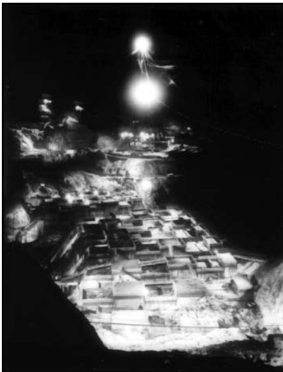
Figure 7-8: Night view of operations at Shasta Dam in 1941, seen from near crest elevation on the left abutment. Source: Bureau of Reclamation.
