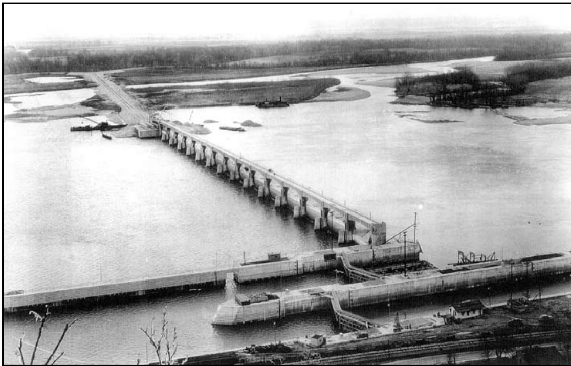
Figure 8-13: Mississippi River Dam #24. Source: Records of the U.S. Army Corps of Engineers, Record Group 77, National Archives and Records Administration, College Park, Maryland..
