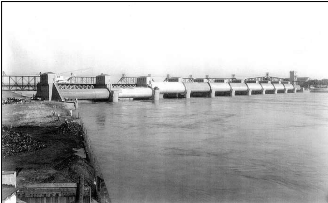
Figure 8-11: Mississippi River Dam #15 showing the roller gates in the raised position on September 23, 1938. Source: Records of the U.S. Army Corps of Engineers, Record Group 77, National Archives and Records Administration, College Park, Maryland.
