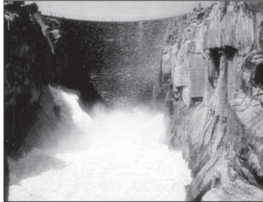
10.5. Pathfinder Dam on the North Platte (Sweetwater) Project.
