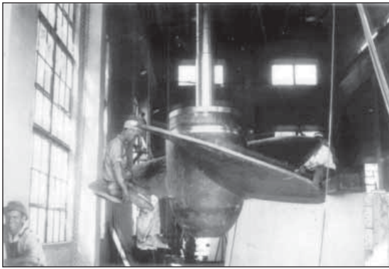
30.4. Bell type 116" turbine runner (Unit 1) at the Siphon Drop Powerplant on the Yuma Project in 1926.
