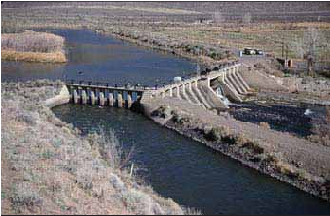
6.2. View of Derby Diversion and Truckee River.
