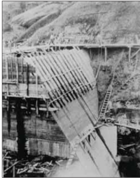
1.7. Construction at East Park Dam, California. Note the vertical formed contraction joint and concrete forms.
