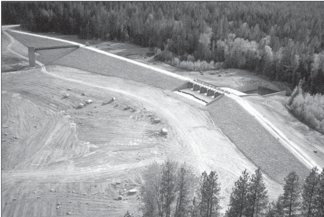
2.22. McDonald Dam: New dam in 2000.
