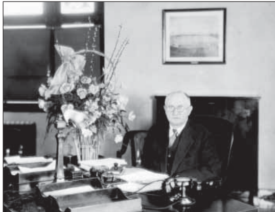
19.3. Commissioner Elwood Mead at his desk in the Interior office building.
