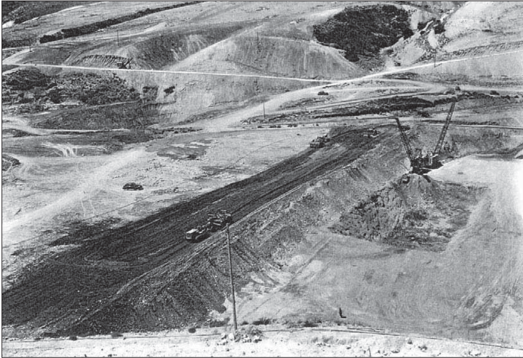
17.4. Construction at Deer Creek Dam.
