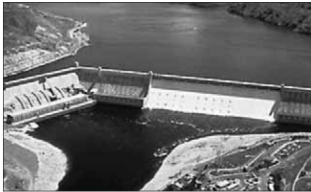
1.31. Grand Coulee Dam, Forebay Dam, and Third Powerplant, Washington.
