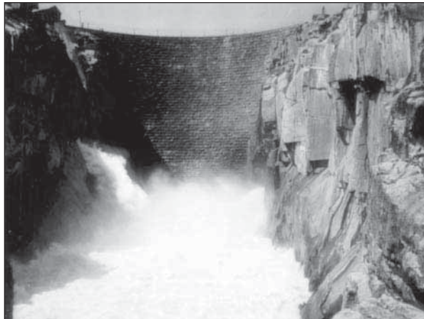
12.3. Pathfinder Dam on the North Platte Project.
