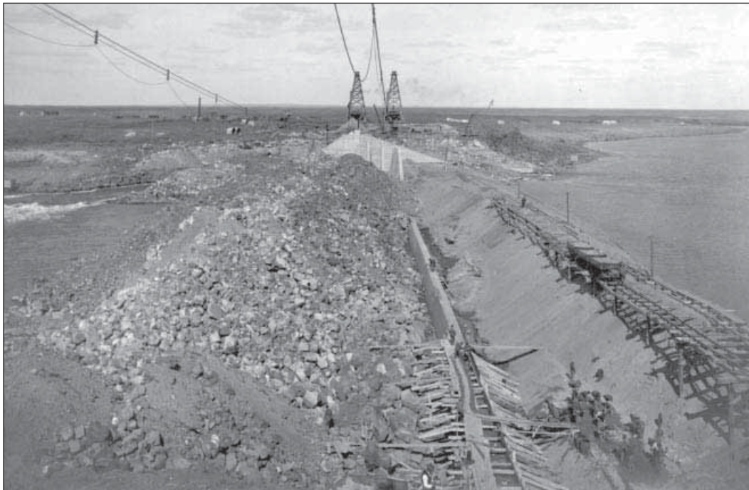
2.4. Minidoka Dam construction.
