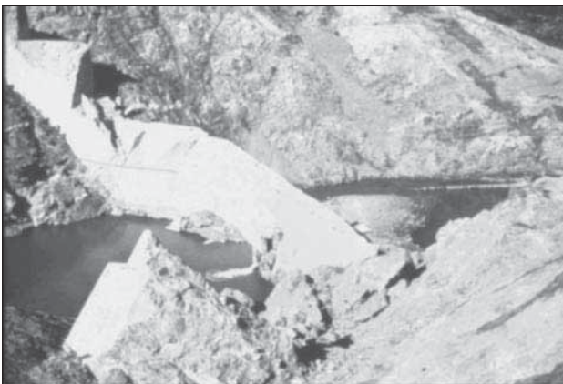
1.40. Malpasset Dam failure, Cannes District, France.
