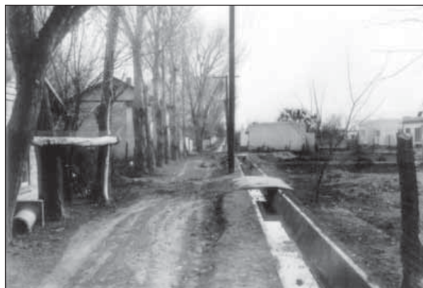
32.3. CCC forces lined small community ditches in Las Cruces, New Mexico, on the Rio Grande Project in 1937.
