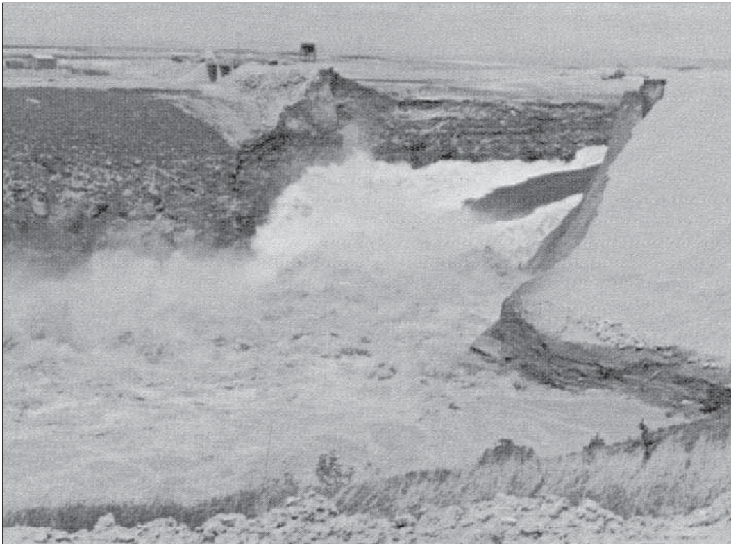
2.17. Teton Dam. Dam completely breached.
