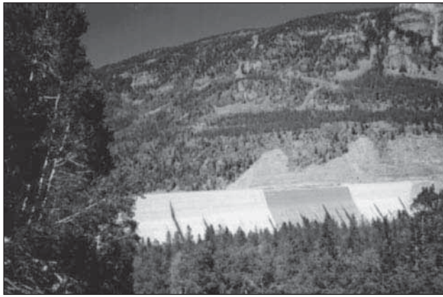
1.51. Upper Stillwater Dam, Utah.
