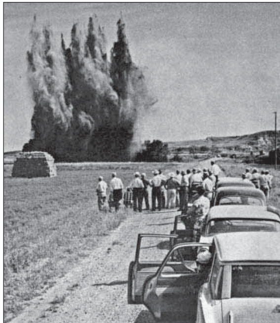
4.4. About 1959 Reclamation experimented with using dynamite to clean drains on the Lower Yellowstone Project.
