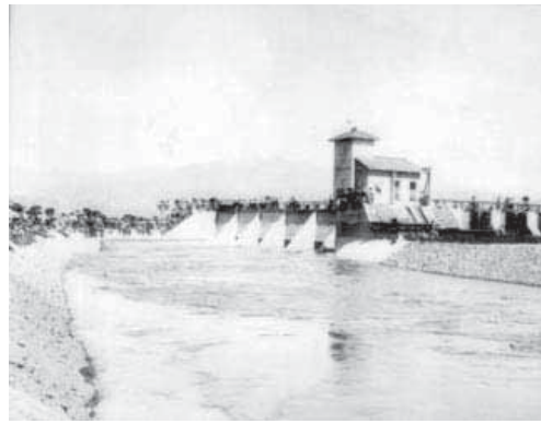
10.6. The Granite Reef Diversion Dam diverting water into the Arizona Canal in 1908.
