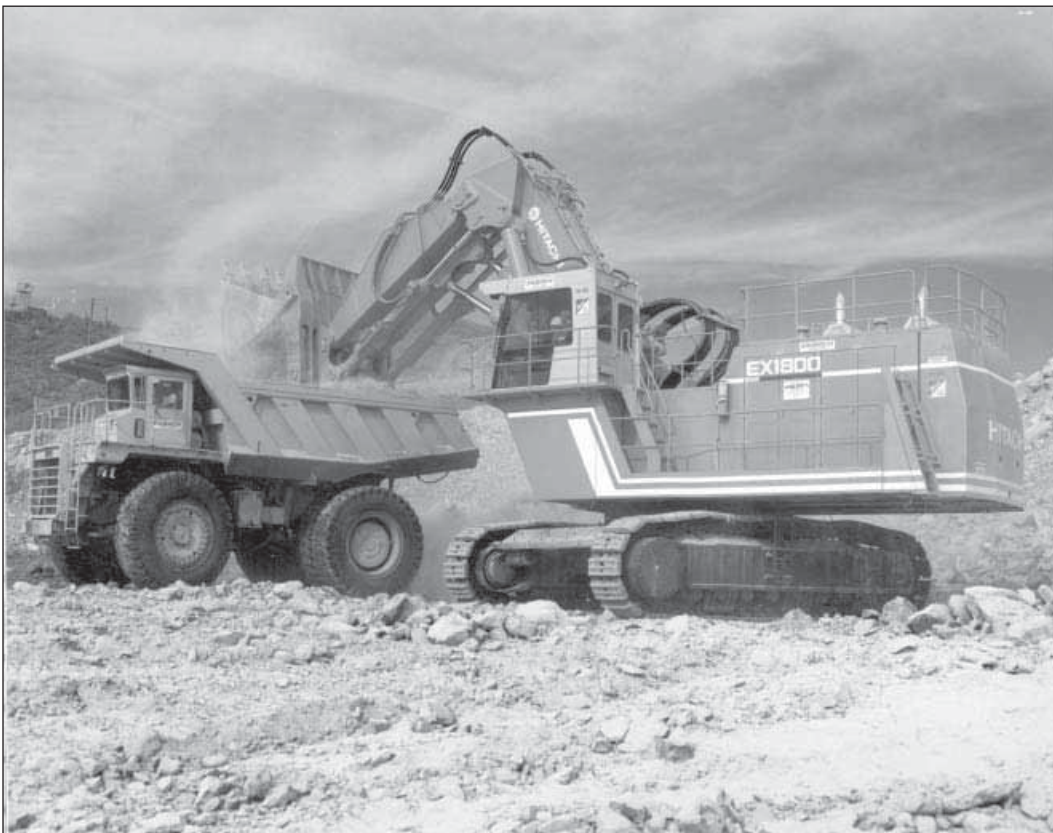
2.24. New Waddell Dam: Construction equipment.
