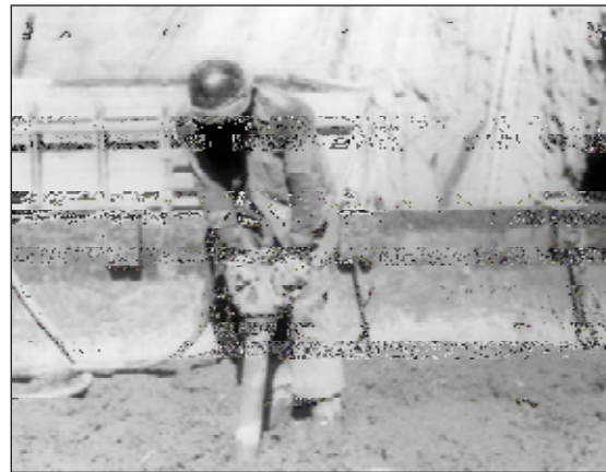
3.7. The use of vibrators allowed a lowered unit water content of the concrete mixture.
