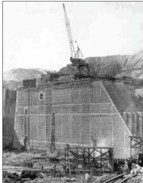
1.33. Construction of Grand Coulee Dam, Washington. (Note Keyed contraction joint.)
