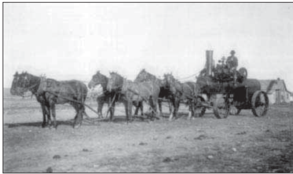
10.4. Freighting a portable engine to a sawmill on lower St. Mary Lake in June of 1906. The lumber was to be used in construction work on the Milk River Project.
