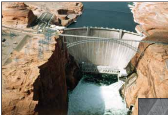
31.4. Glen Canyon Dam and Powerhouse.
