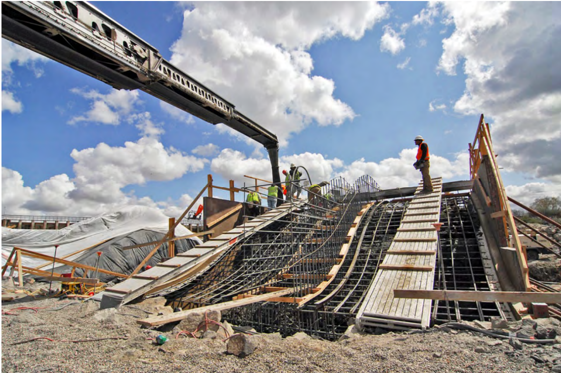
Minidoka Dam Spillway, Minidoka Project, Pacific Northwest Region.
