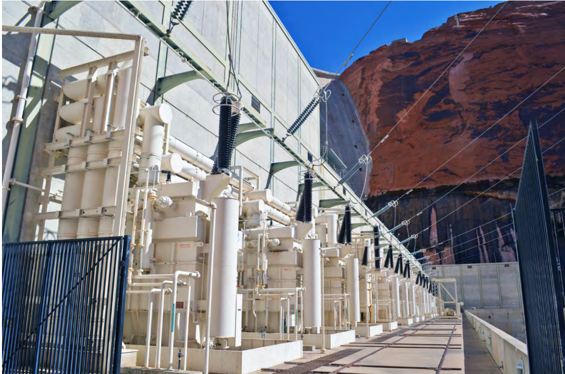
Glen Canyon Dam, Colorado River Storage Project, Upper Colorado Region.
