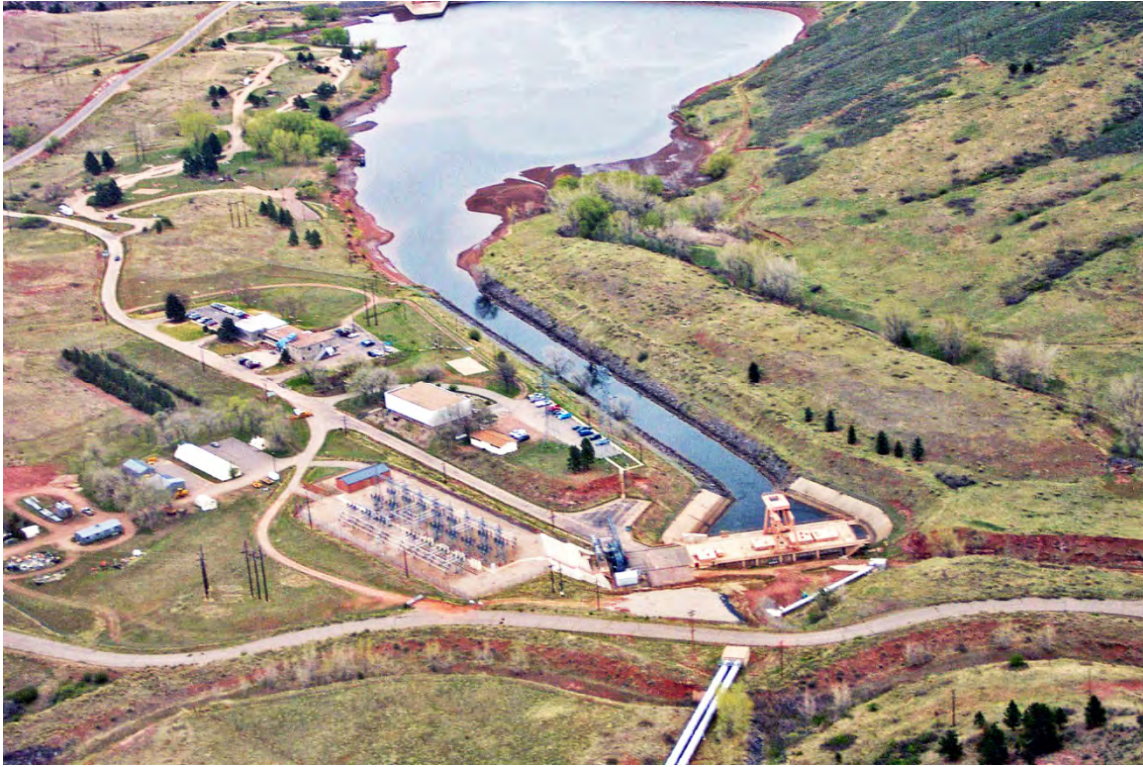
Flatiron Powerplant, Eastern Colorado Area Office, Great Plains Region.
