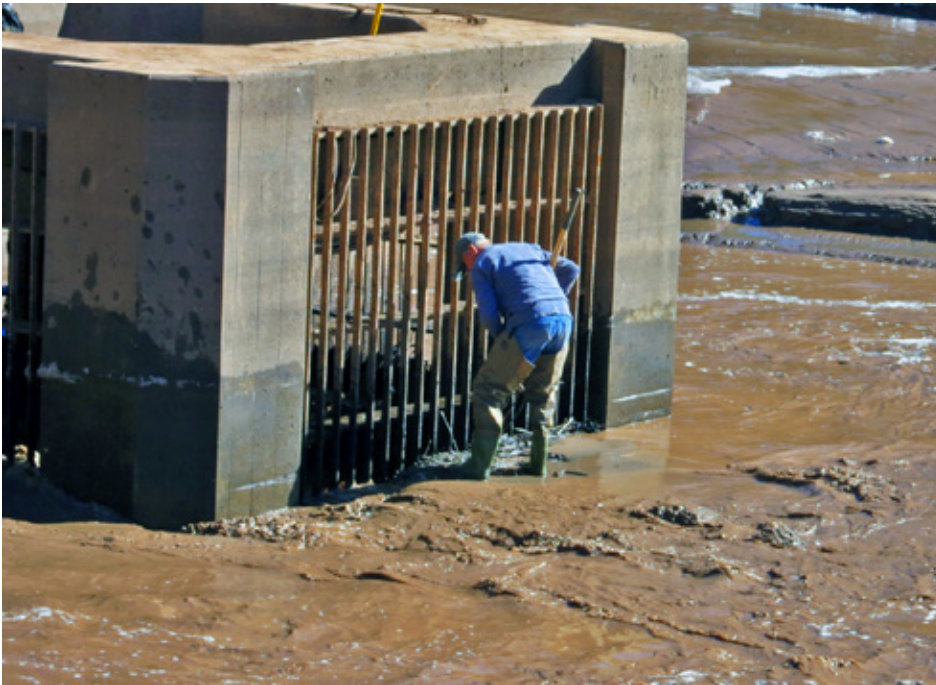
Paonia Outlet structure during emergency actions to maintain diversion, November 11, 2014.
