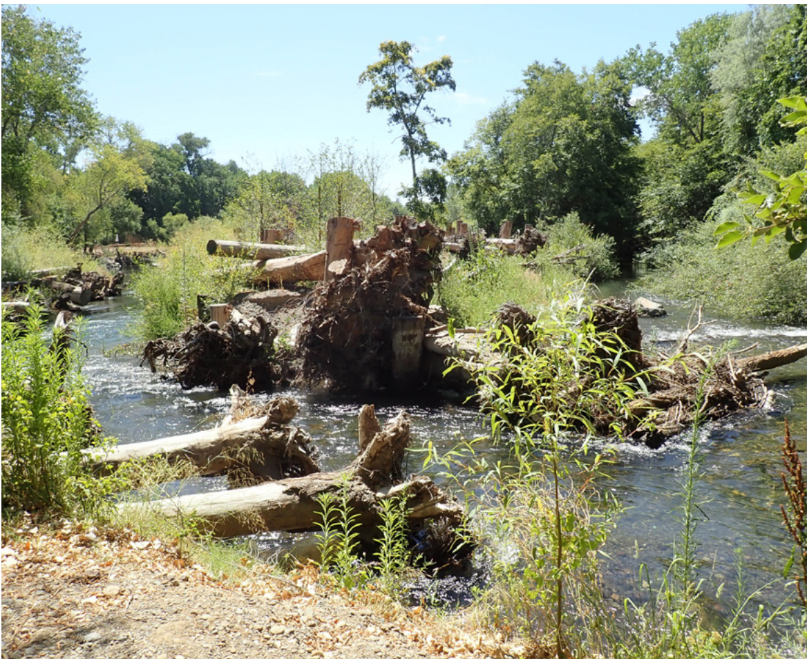
LWS installations on Dry Creek near Healdsburg, California.
