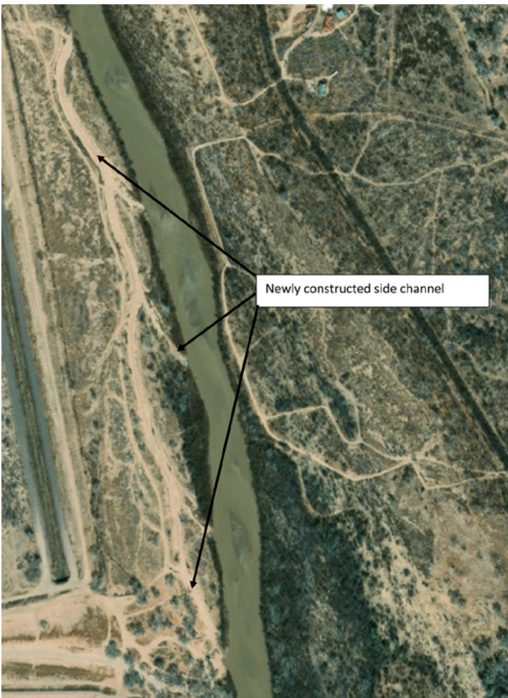
Newly constructed habitat features that includes several connections to the main channel.
