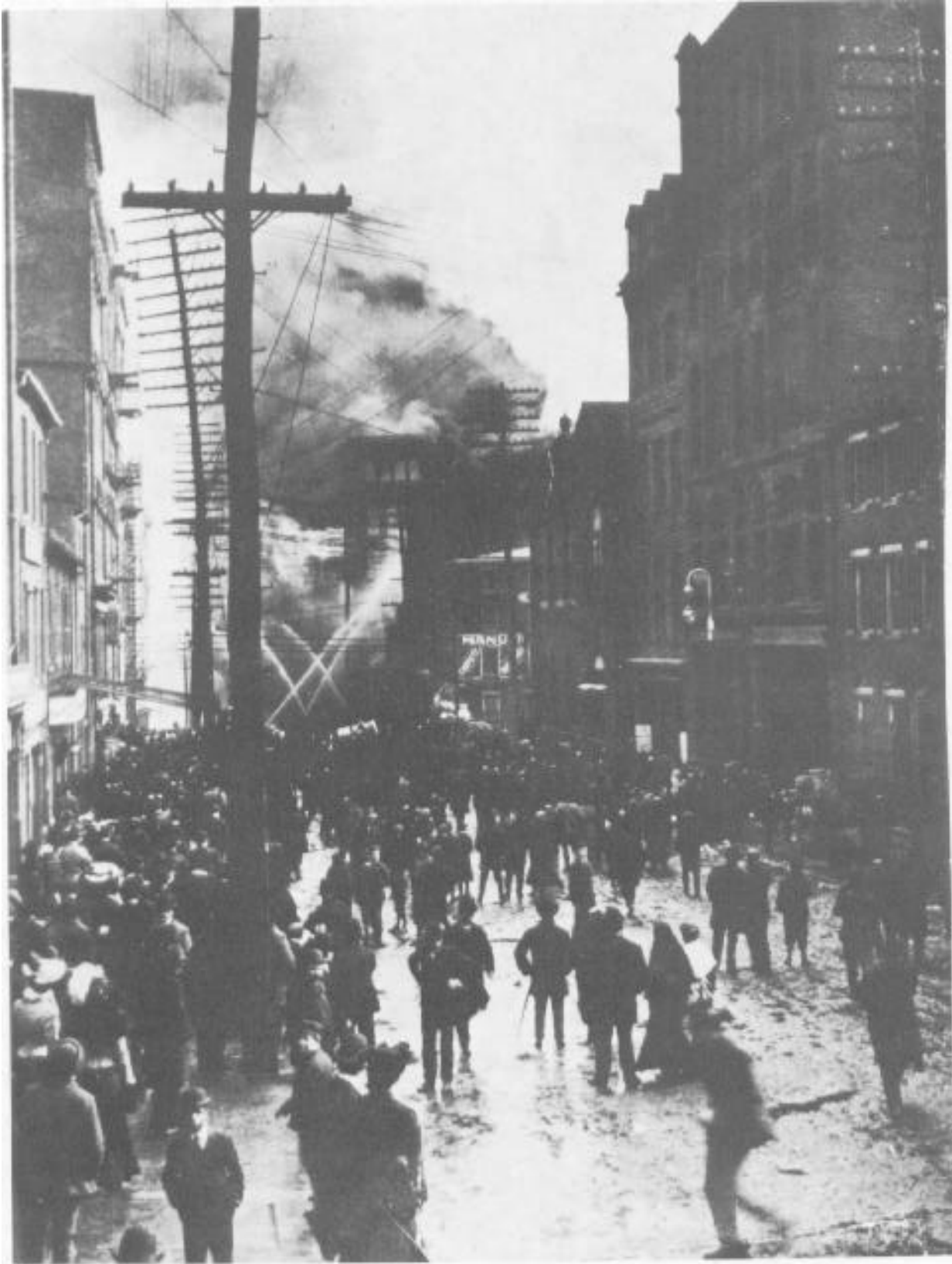
Major turn-of-the-century fires, such as Baltimore's in 1904, aroused concern about fire safety in buildings.
