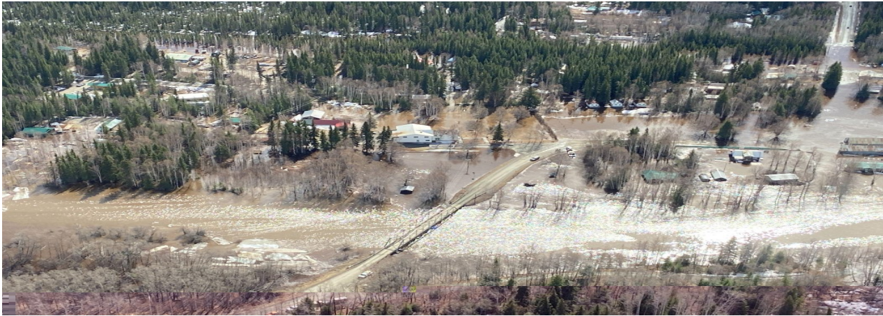
Fig 3: Many buildings in the community had water in or around them. The bridge over Manley Slough was within six inches of being overtopped.
