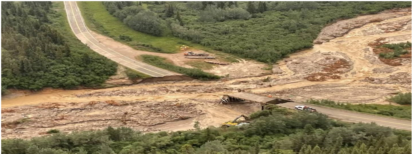
Fig 15: Washout at Bear Creek at Milepost 223 on the Richardson Highway (courtesy Alyeska Pipeline)
