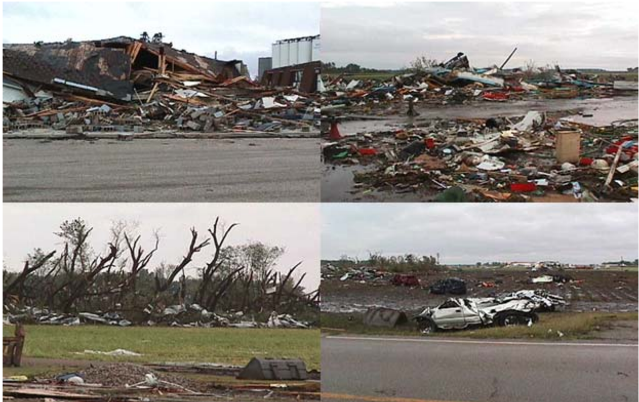
Figure 3. Photographs taken by a National Weather Service storm survey team, showing tornado damage up to EF4 intensity in Northwood, North Dakota.
