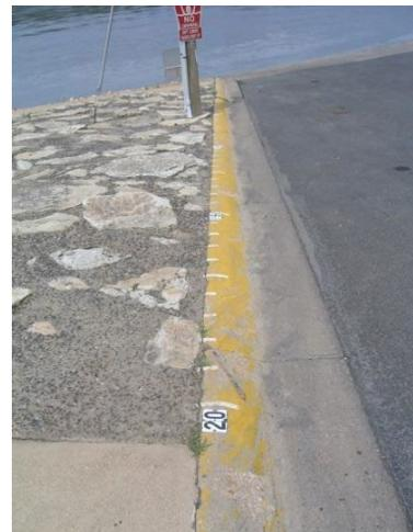
On some rivers, especially where man-made structures such as bridges are rare and where vertical or staff gauges can be damaged by ice jams and breakup, profile gauges are used. These consist of a marker, usually a metal strip several inches wide, or a bright painted stripe along an existing concrete or asphalt surface, which extends down toward the water.
