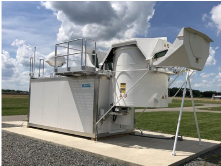
Figure B-1: Automated Radiosonde Observing System (AROS / Autosonde / AS15)
