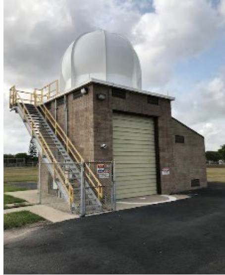
Figure B-15: High Bay
