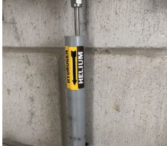
Figure K-9: Acceptable Markings for Helium/Hydrogen Tubing
