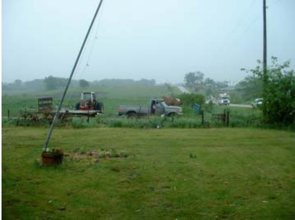
Pole leaning southeast
