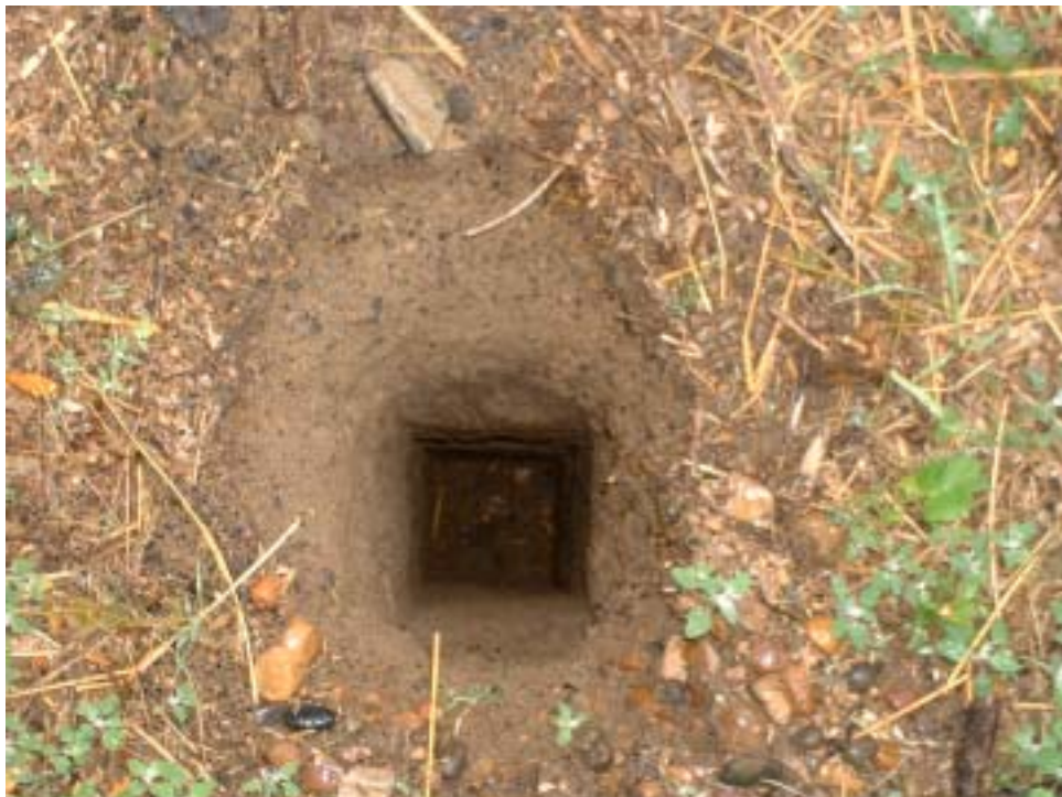
Hole left over after pole was removed by wind
