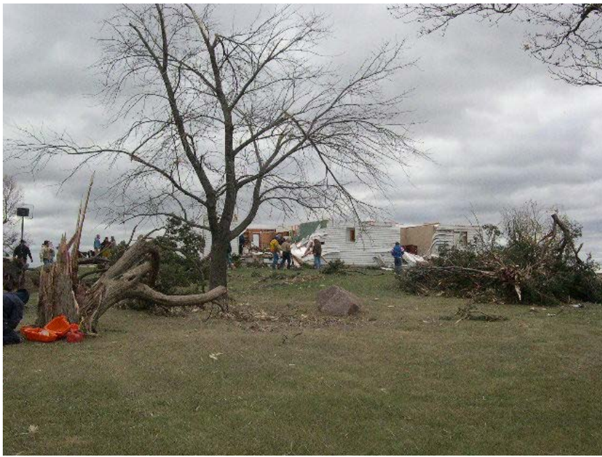
Home heavily damaged near 6 Avenue north of Pilot Mound in Webster county.
