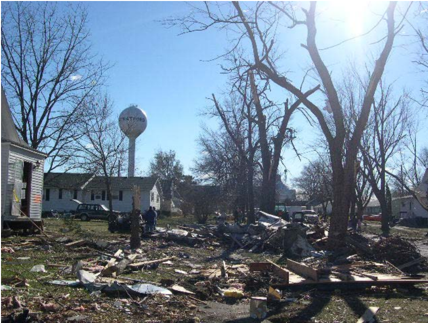
Debris accumulating from heavily damaged homes in Stratford.
