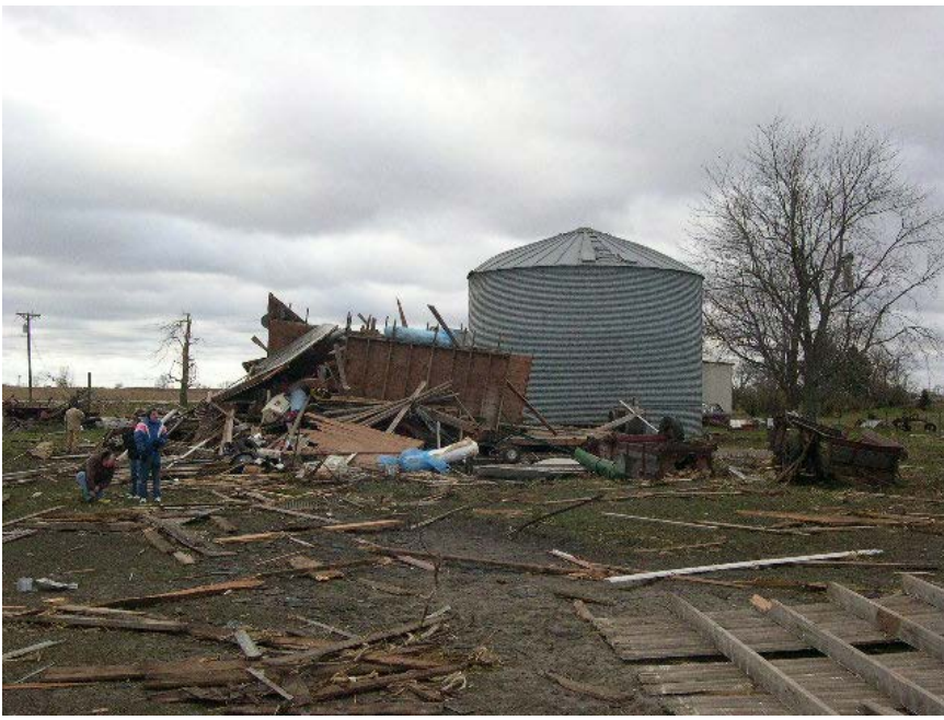
Damage to outbuilding and grain bin near E18/US 169 in Boone county.
