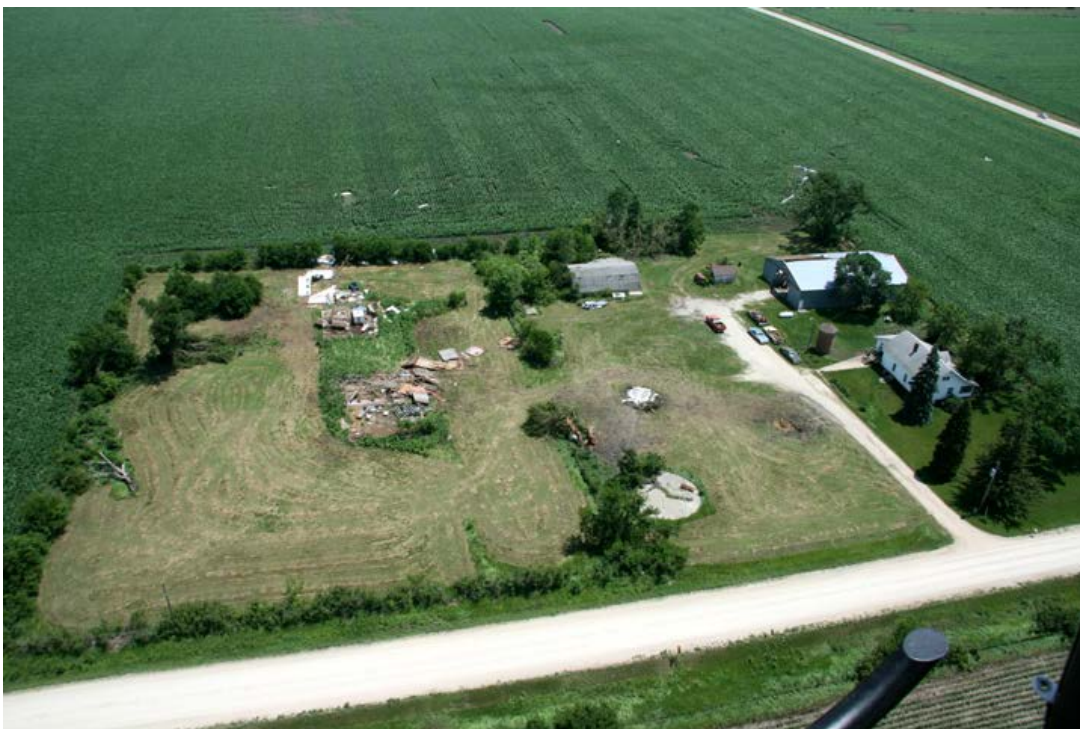
Tornado damage west of Cumming just east of I35. Courtesy IowaHelicopter.com
