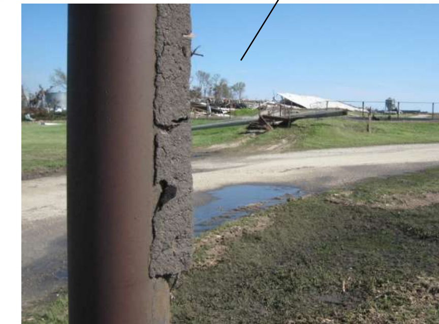
Mud splattered houses and poles were common WNW of Dunkerton, with most out-buildings flattened. This damage was in the EF1-2 range. NWS survey team photo.
