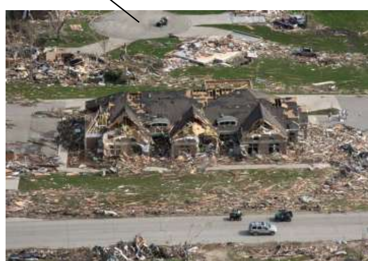
The most severe destruction in Parkersburg occurred south of the tornado core, which tracked directly over the First State Bank (left photo). Several fatalities occurred in the neighborhood of the center photo, as floors were swept away exposing basements. Mature trees were reduced to debarked stubs. The high school (right photo, Getty Images) received EF2-3 damage.
