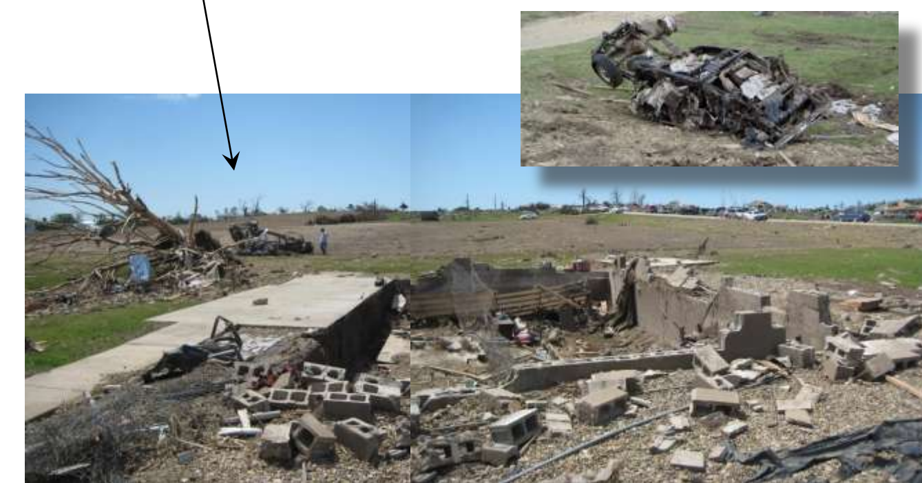
North of New Hartford, a woman was killed as her home was swept away. Only vehicle frames and tree trunks remained. Even the basement was cleared. The tornado was rated EF-5 at this location. The New Hartford cemetery is in the background. NWS survey photos.
