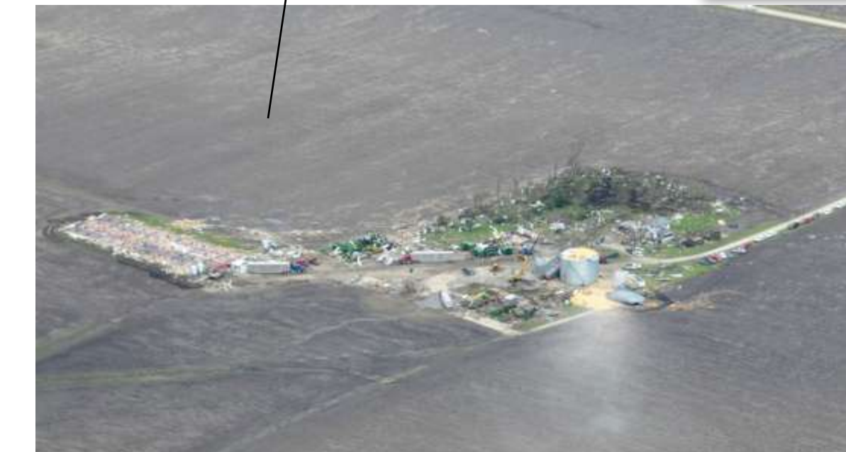
Damage on Lester Rd northwest of Dunkerton approached EF3 at several farm sites. Many hog confinement buildings were flattened. Here, hogs can still be seen in the building with some being loaded onto trucks. Civil Air Patrol photo.
