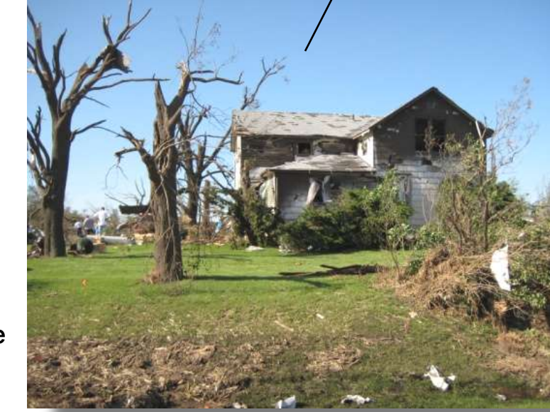
Mud splattered houses and poles were common WNW of Dunkerton, with most out-buildings flattened. This damage was in the EF1-2 range. NWS survey team photo.
