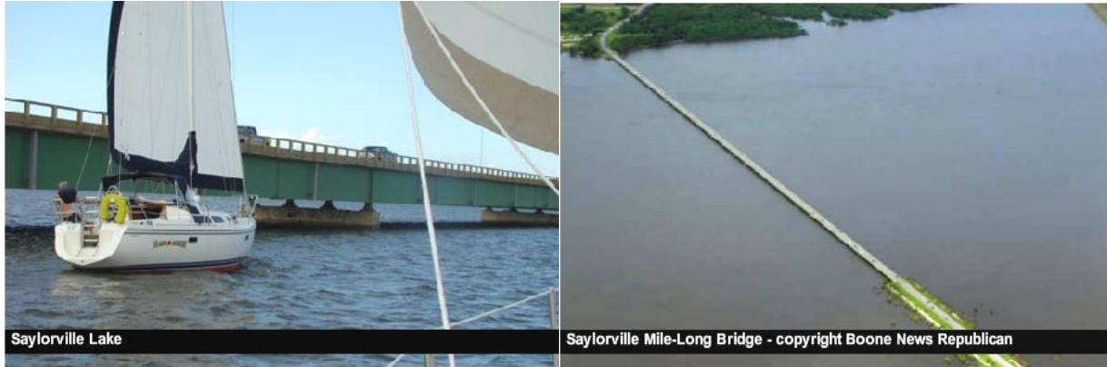
Figures 7 (left) and 8 (right): Saylorville Lake and the Mile-Long Bridge (State Highway 415 to Polk City, IA) during the week of June 12 th 2008. Photos are courtesy Iowa Department of Transportation and Boone News Republican.
