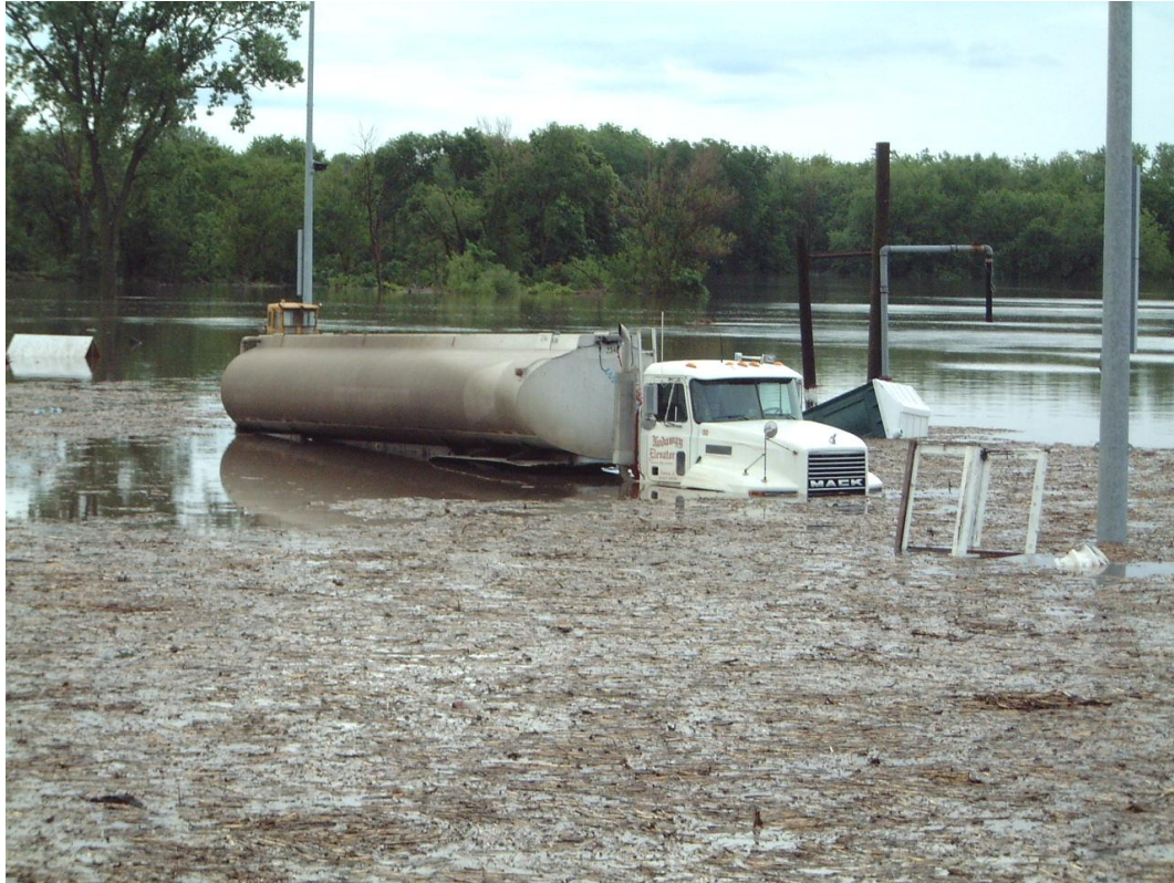
Figure 30: Flooding near the Adams County Speedway in the city of Corning. Photo Courtesy of Bob Simon.
