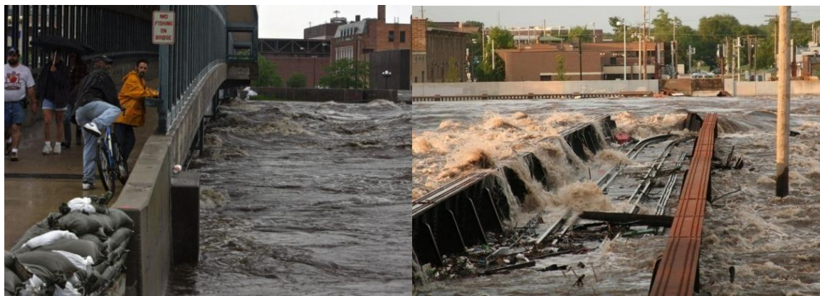
Figure 13 (left): Cedar River in Waterloo, IA on June 11, 2008. Photo is taken by Associated Press David K. Purdy.
