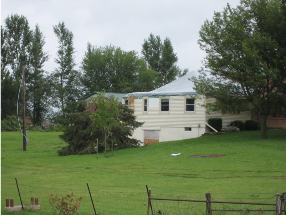
Figure 2. Damage to the roof and siding of a house north of West Euclid Avenue.
