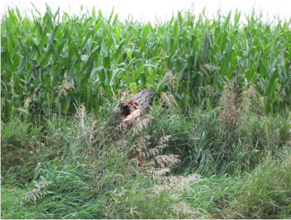
Figure 6. Power line pole snapped off along 90th Avenue.
