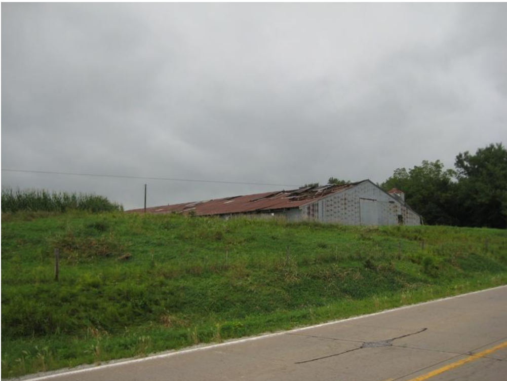
Figure 5. Damage to a metal storage building along County Highway R57.
