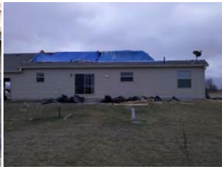
House with partial roof removal. Photo by NWS Des Moines, Iowa.
