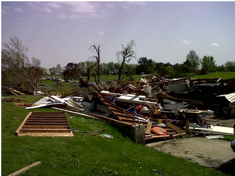
A one-story residence sustained major damage just west of Creston.
