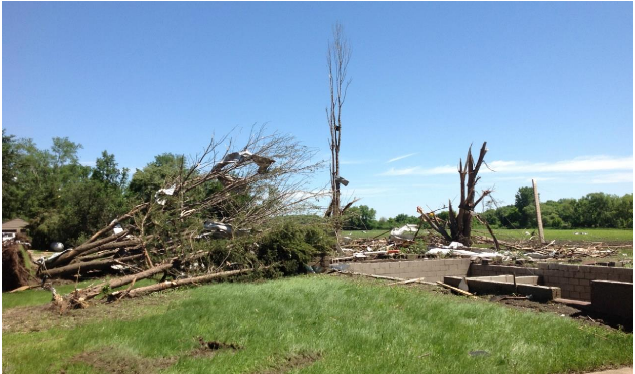
An older house was detached from its cinder block foundation and destroyed on the north side of Belmond. Many trees were uprooted and flattened in this area as well.
