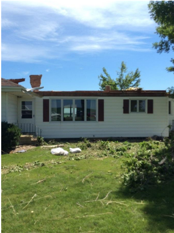
Two houses early in the tornado's track sustained roof damage.
