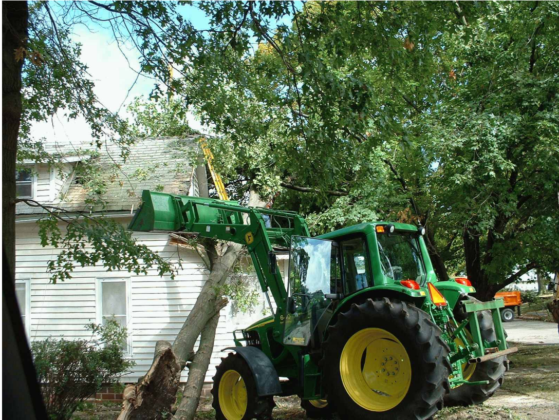
A large tree blown on to a house in central Creston.
