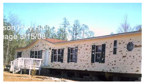
Fig. 9. Another major hazard associated with downbursts is from wind-driven large hail, which can cause injury and major property damage, such as with this manufactured home. Photo courtesy of Greenwood County Emergency Management.
