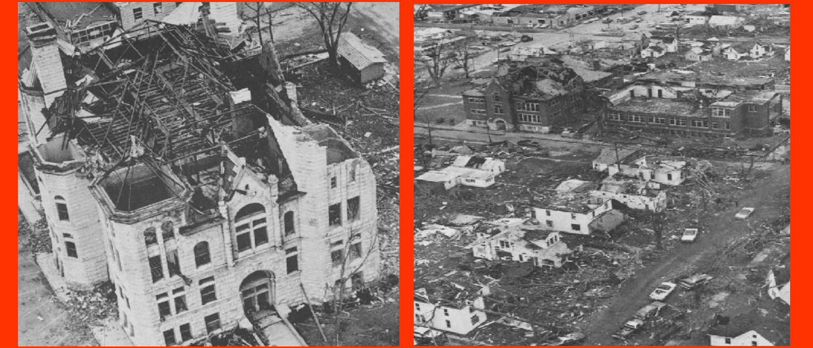
Tornado damage at the Monticello court house (left) and throughout the town of Monticello, IN (right).
