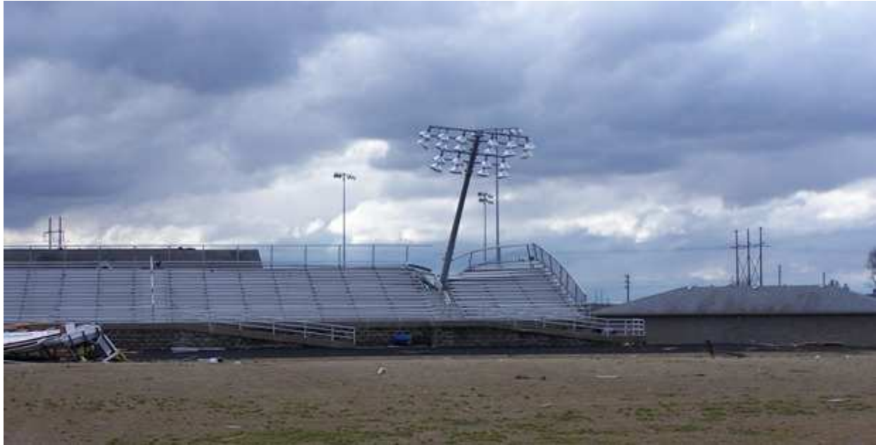
Tornado damage in Elizabethtown, Kentucky, on February 5. Photo: NWS
