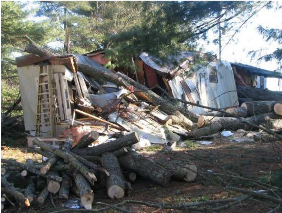
Tornado destruction near Henryville, Indiana on January 29. Photo: NWS
