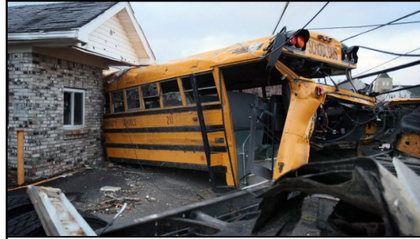
An EF4 tornado struck Henryville, IN (Clark Co.) on March 2, 2012. Safe rooms offer "near-absolute protection" during these devastating events.
