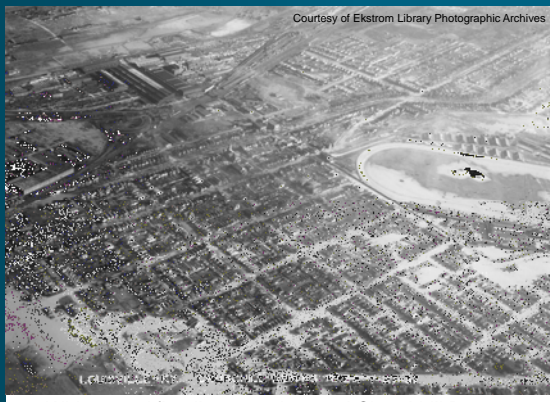
Widespread flooding at and around Church Hill Downs.
