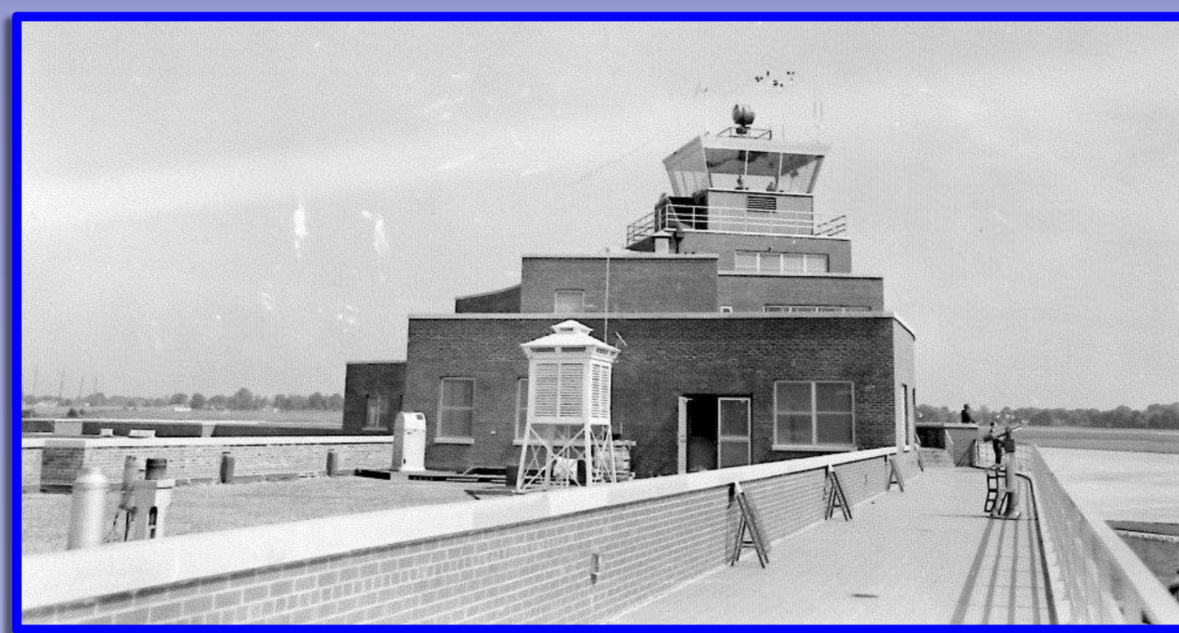
Meteorological instruments on the roof of the terminal building at Standiford Field in the late 1960s.
