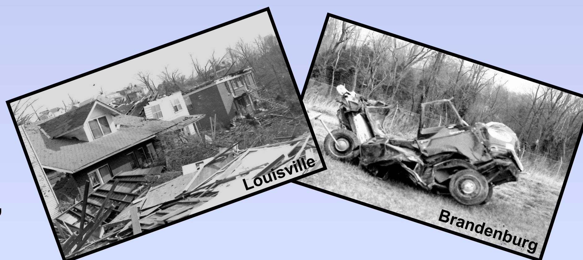
On April 3, 1974 a tornado touched down just half a mile from the weather office and grew to F4 strength as it plowed through northeastern Louisville and into Oldham County. The weather office was battered by 84 mph winds, knocking over the meteorological instruments that were on the office's roof.
