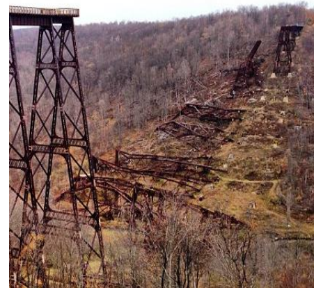
It only took an EF-1 tornado to destroy this structurally unsound bridge in Pennsylvania.
