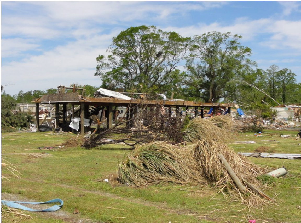
Damage from EF-3 tornado in Beaufort County, April 25, 2014
