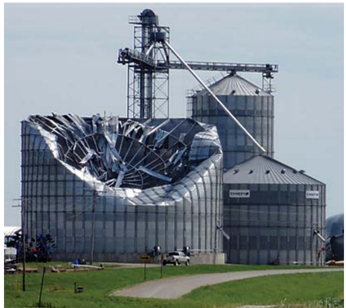
After a tornado, watch out for dangerous debris, such as sharp metal, glass, or downed power lines.. Photo: NOAA
