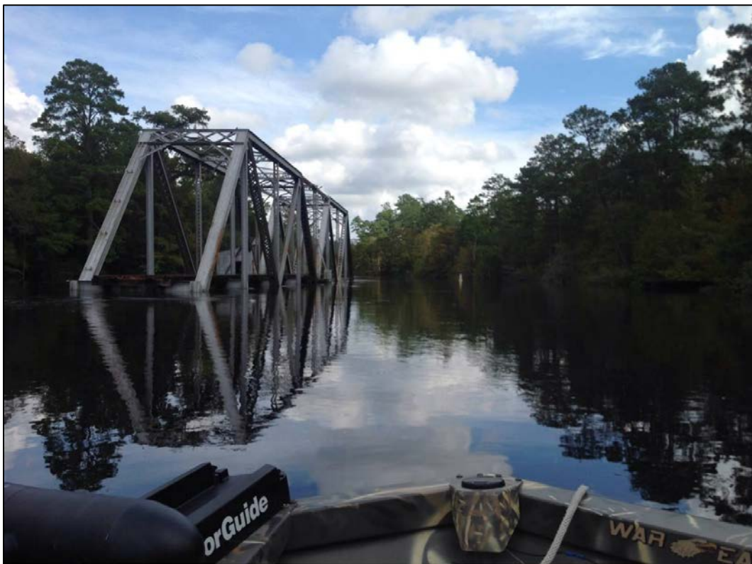
Figure 13: Waccamaw River Floods out Railroad Bridge Flooded in Conway, SC. Source: USGS
