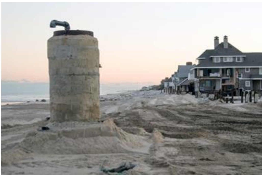
Figure 12: Mantoloking, N.J., November 5, 2012. Drainpipe shows the pre-storm height of sand dunes. Source: Liz Roll, FEMA
