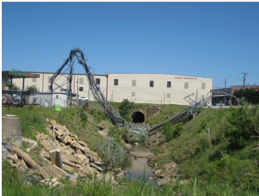
Figure 7: Destroyed NWR transmitter tower at Cullman, AL (courtesy of WFO Huntsville, AL)
