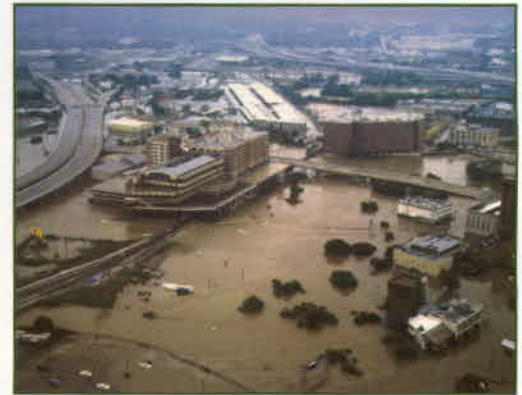
▲ Photo: Harris County Flood Control District, Houston, Texas
