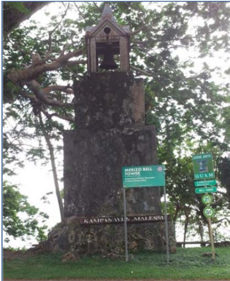
Merizo Bell Tower.
