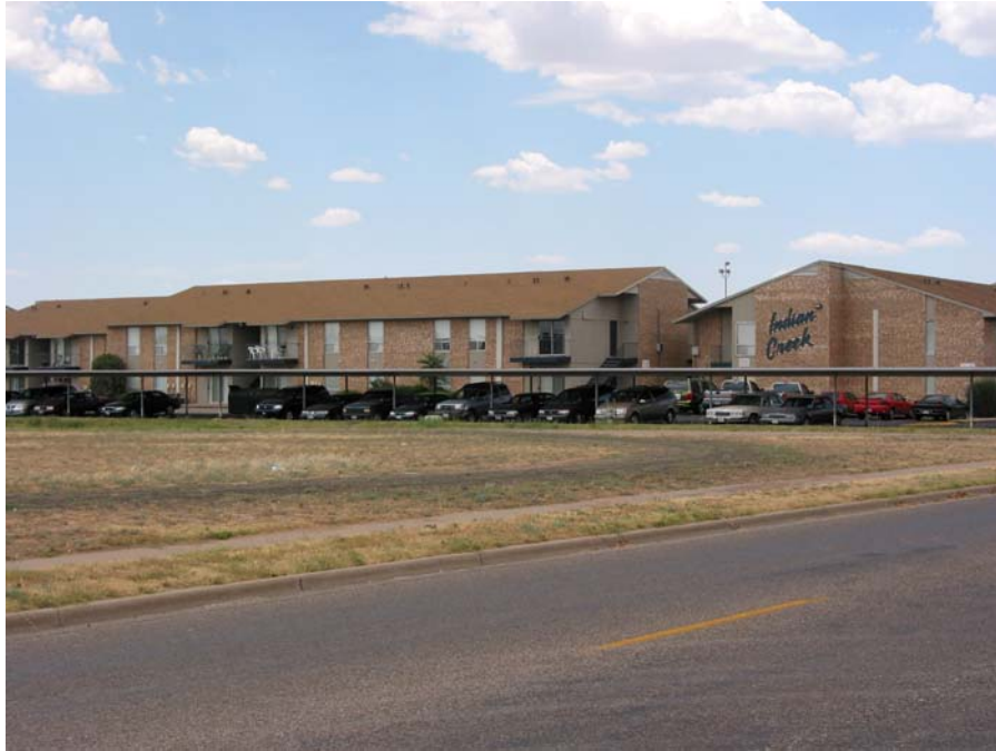
ACT: Gable roof, asphalt shingles, wood decking, light-framed wood construction, brick veneer, wood stud walls, balconies
