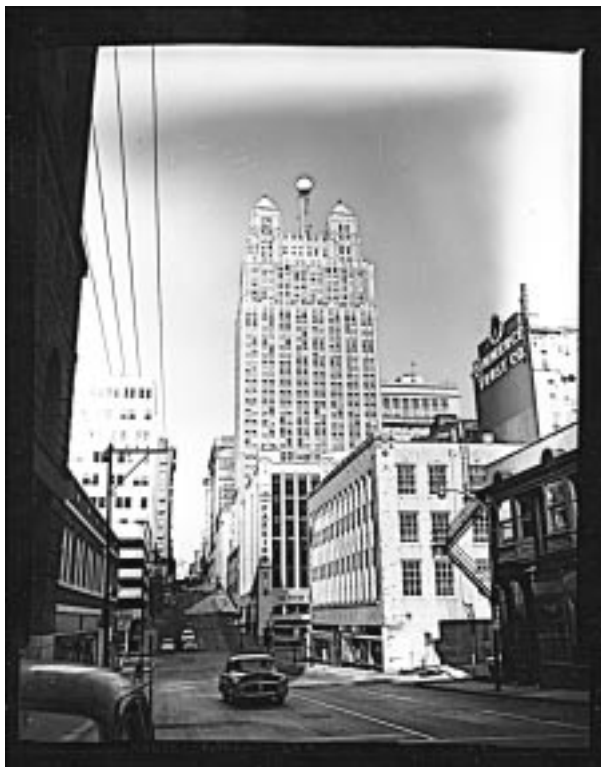
FIG. 8. Federal building at 911 Walnut Street, Kansas City, MO, c. 1958.
