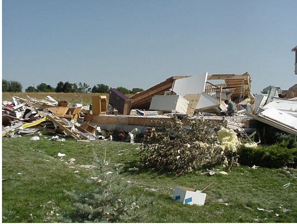
Figure 7b: Closer image of the home in the lower left of Figure 7a showing walls down, but the debris is not far from the house. Pictures courtesy of the NWS Office in Wilmington, OH.
