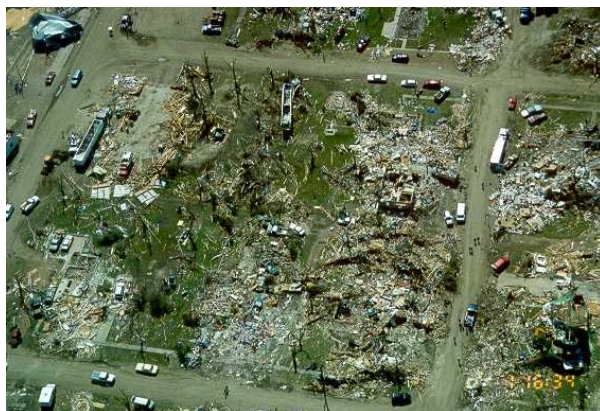
Figure 9: Aerial view of damage from the Spencer, SD tornado, May 30, 1998. Photo courtesy of Brian Smith.
