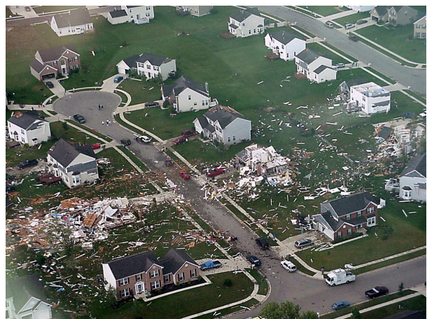
Figure 7a: Aerial view of damage from the Xenia, OH tornado, September 20, 2000.
