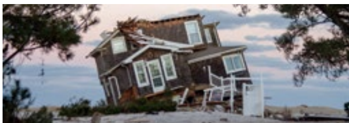
Mantoloking, N.J., Nov. 5, 2012 - This house was destroyed by the storm surge of Hurricane Sandy. FEMA
