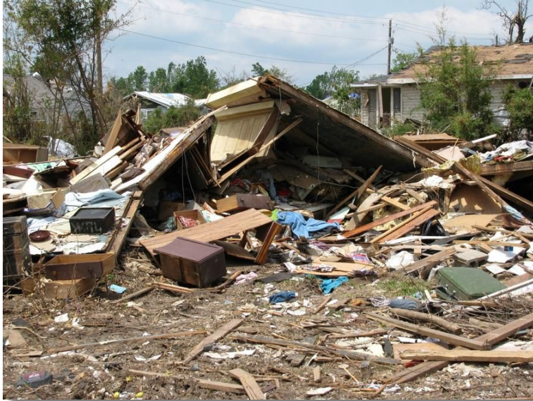
A destroyed wood frame house in Concord, AL
